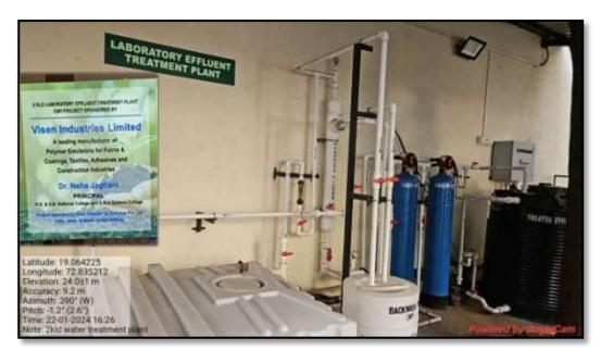
Liquid from Biology & biotechnology laboratories are channeled to a tank designed based on **Phytorid technology, patented by NEERI**.
