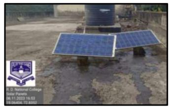
Two solar panels in North -west direction on the College Terrace installed by the Department of Physics connected in series with output of 160 watts per hour and storing capacity of 24 volts.
